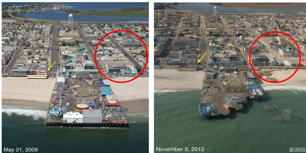
Figure 2. Before and After Hurricane Sandy Storm Damages (Seaside Heights, NJ).
