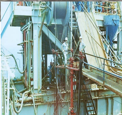
Platform with a drilling rig and a well, James “Cecil” Broussard (2002)
