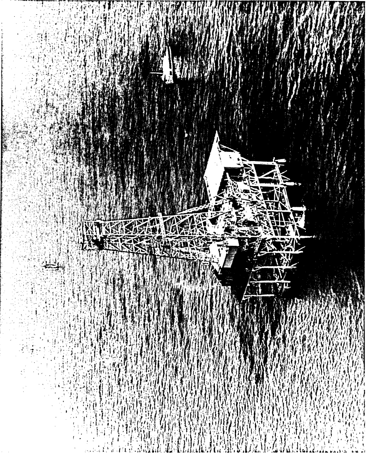
FIGURE I-9 SELF-CONTAINED FIXED PLATFORM
