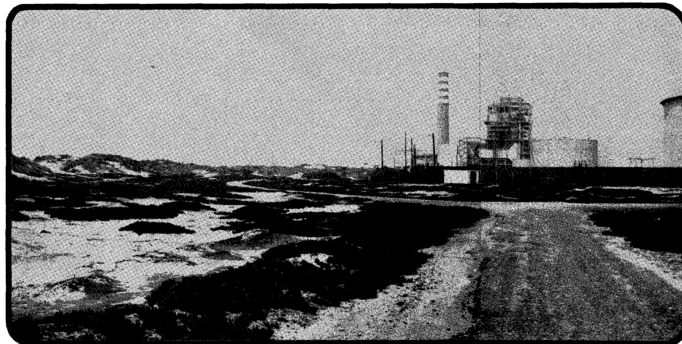
VIEW TOWARD NORTHWEST FROM SOUTH OF SITE
