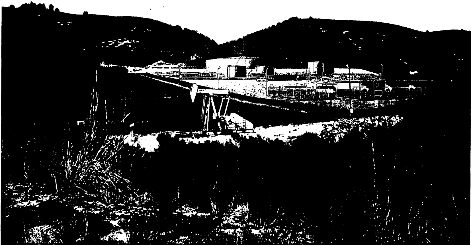
Figure 5.9-3 Simulation showing proposed Lompoc Dehydration Facility immediately after construction, seen from viewing position #1, northbound lane.
