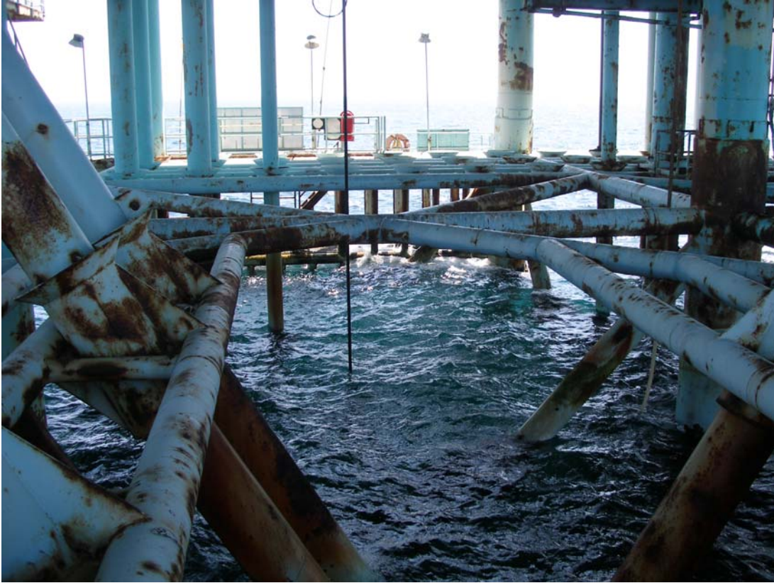
Figure 18. The 15-foot deck of platform C showing central work area.
