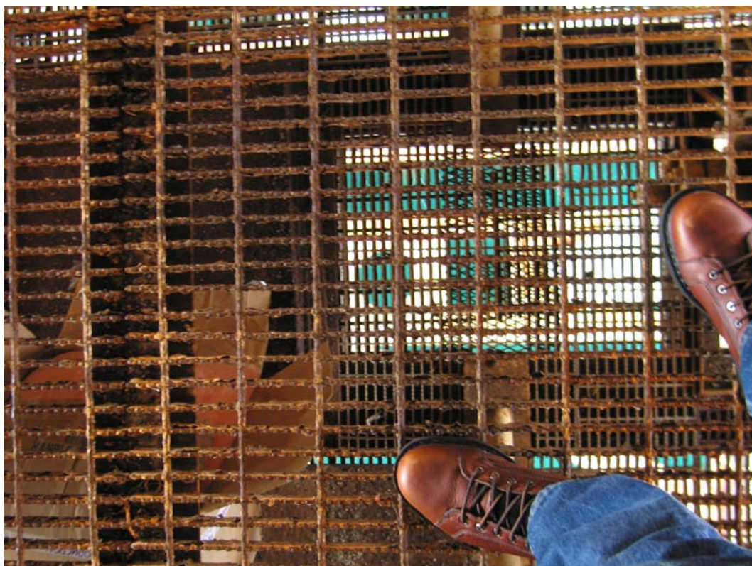
Figure 9. Open well slot and openings through all three decks
