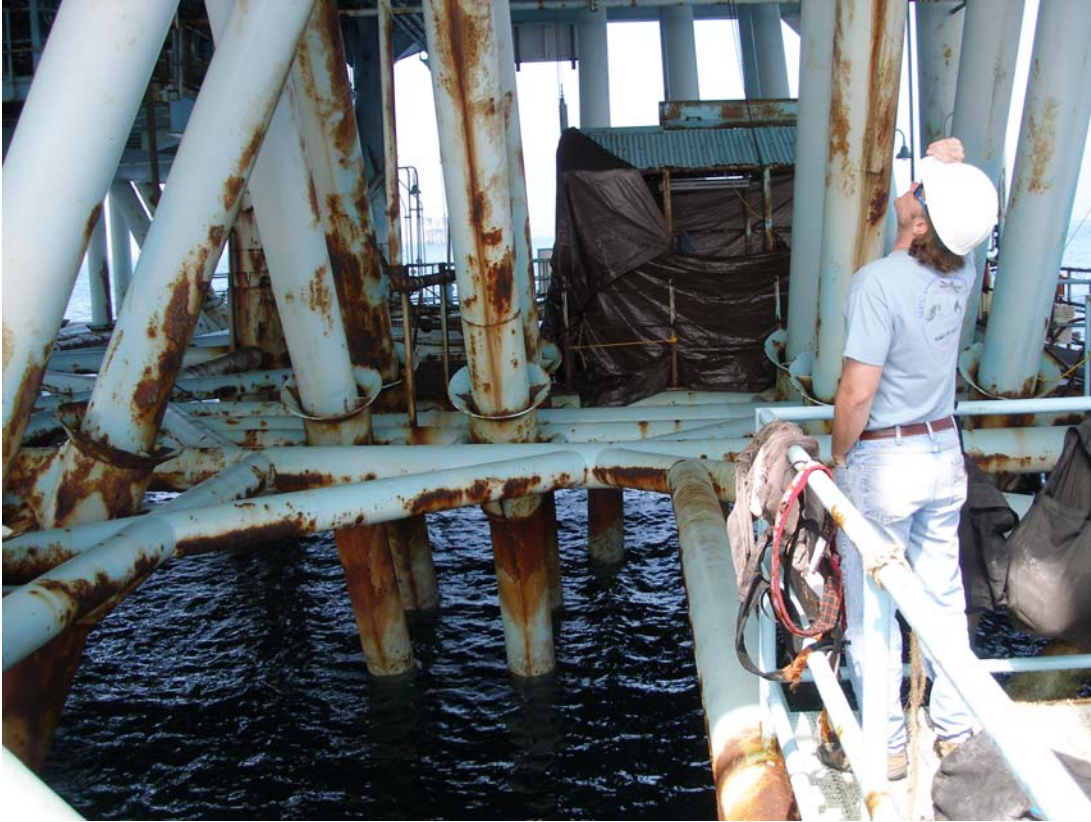
Figure 14. 15-foot deck on platform A with central work deck.
