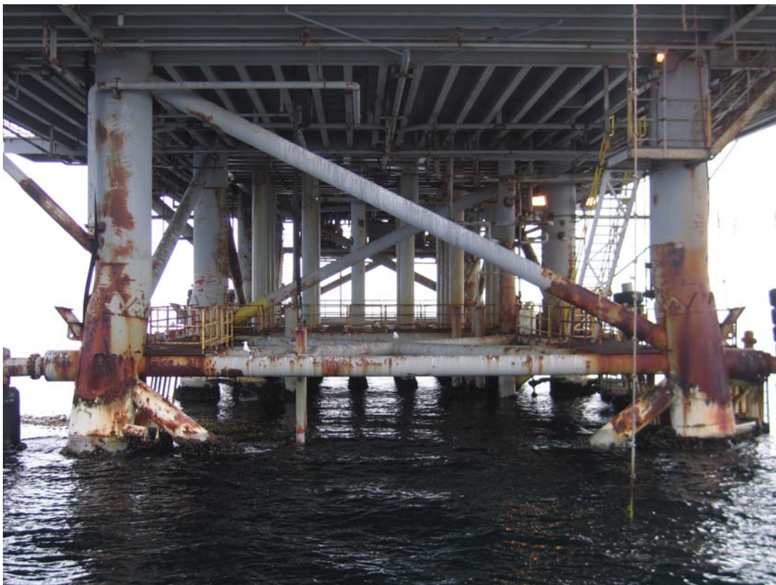
Figure 3. 15-foot deck with conductors
