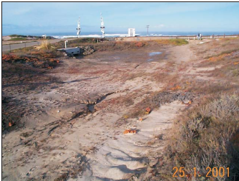
Figures 5.4-2: Example of a Catchment Basin (Basin 1) Adjacent to Onshore Portion of the Pipeline Route. (A weired Concrete Outlet is Shown Near the Upper Left Corner of the Photograph.)
