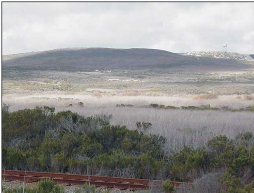
Figures 5.13-6: Route 246 to Valve Site #2 (View Position 5) (View of Surf Substation looking west from the west end of Ocean Avenue. The low vegetation is in the foreground, the substation is in the mid-ground and the ocean is in the background.)
