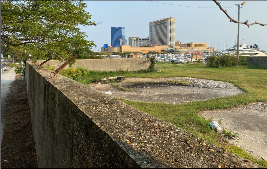
Photograph 2. Overview of the southern portion of the proposed Facility Site, enclosed in a concrete wall with roughly octagonal concrete foundation pads. View to the north.
