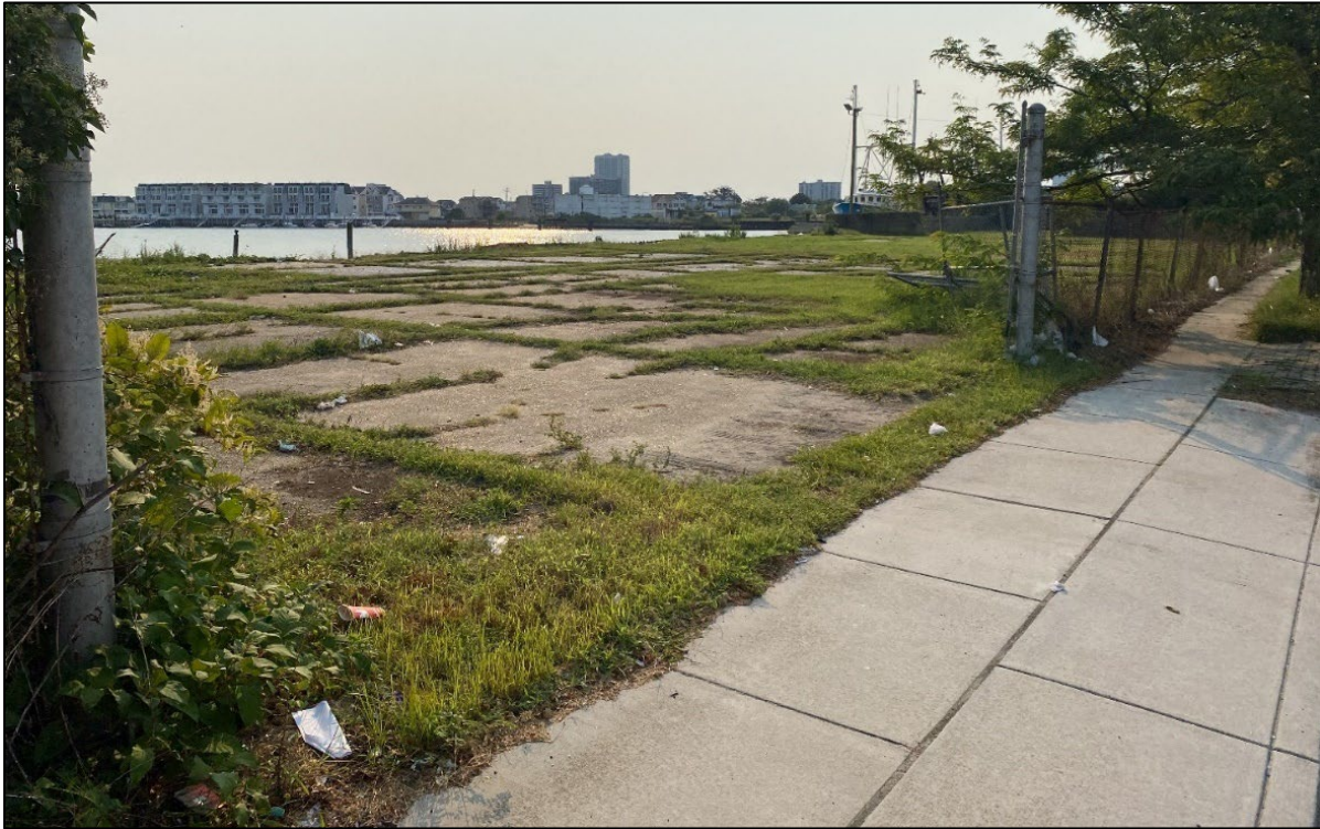
Photograph 1. Overview of the shoreside parcel at 801 North Maryland Avenue with cracked concrete paving and chain link fence. View to the southeast.
