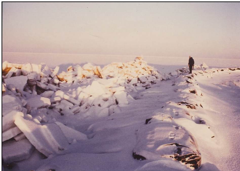
Figure 2.4-6 Ice Rubble Pile 6 m High Formed on West Side of the Duck Island 3 Manmade Gravel Island during a 20-kt Westerly Storm on 15-17 October 1984
