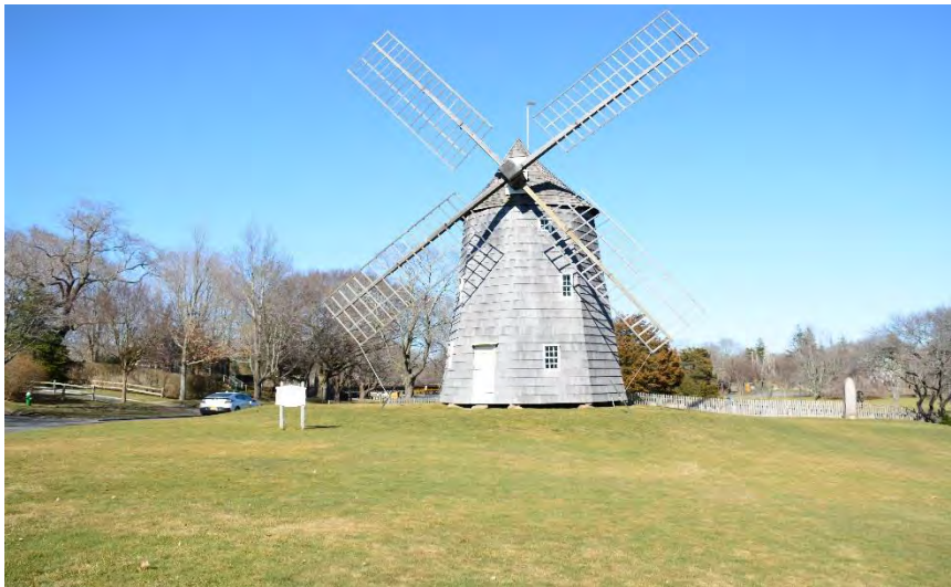
Inset 12 – NRHP-listed Hook Windmill within North Main Street Historic District
