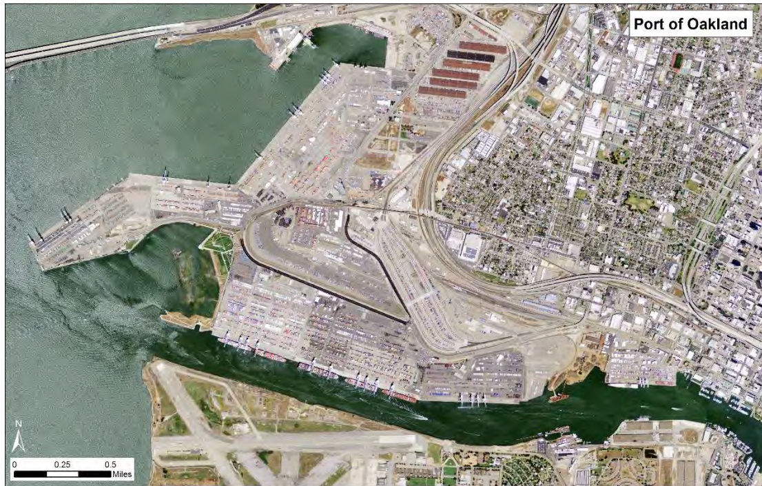
Figure A-5. Port of Oakland
