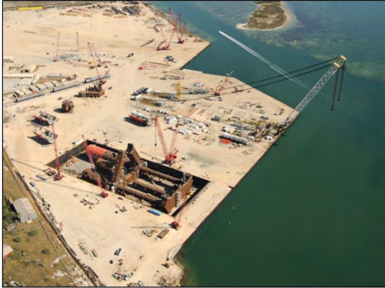
Figure 4-8. Gulf Island Fabrication Company, Ingleside, Texas. (Center for Land Use Interpretation 2016)
