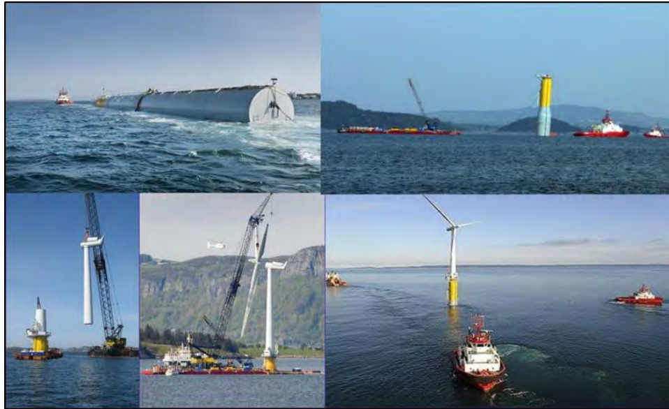
Figure 3-4. Spar demonstration project installation example (Hywind 2015)
