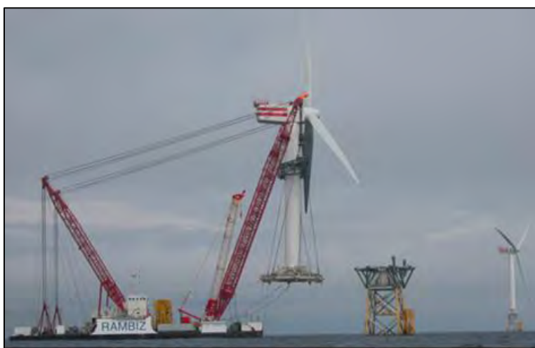
Figure 3-2. Floating Crane Barge Rambiz 3000 installing a wind turbine (Wind Energy The Facts, 2016).
