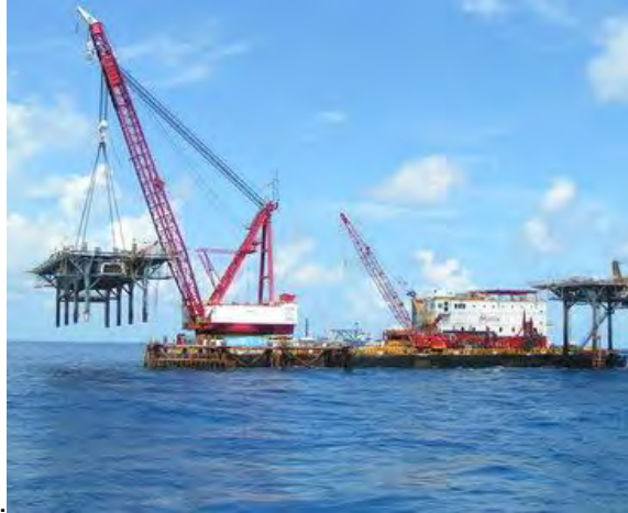
Crane Barge (1000+ ton) 17 Floating Crane E.P Paup [ http://www.mansonconstruction.com/ep-paup/ ]
