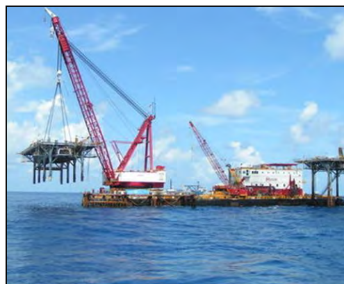
Figure 3-10. Floating cranes, Manson 1000 ton E.P. Paup (Manson, 2015)
