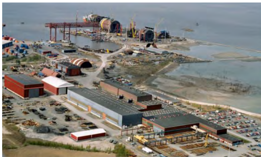
Figure 4-3. Hywind construction location in Pori, Finland (Technip 2013)
