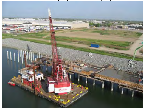
Crane Barge (700-1000 ton) 16 Manson Crane
