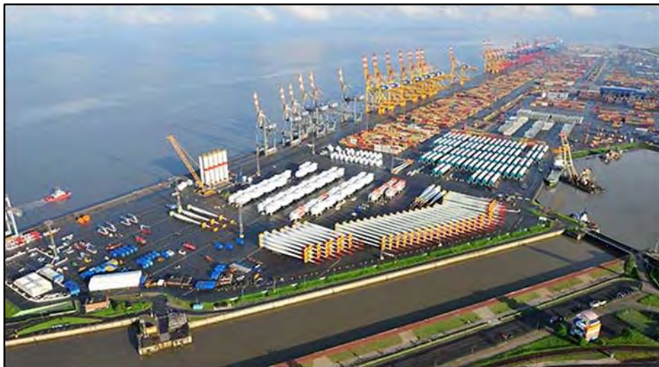
Figure 2-9. Example offshore wind (fixed foundation) Cluster Port in Bremerhaven, Germany (Eurogate 2015)
