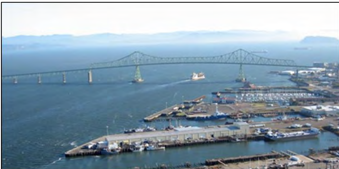
Figure 5-1. Port of Astoria and Astoria Bridge (Longshore Shipping News 2012)
