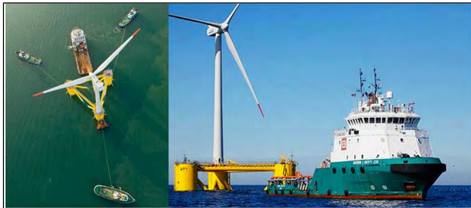
Figure 3-3. Semi-Sub demonstration project installation (WindFloat, 2014)
