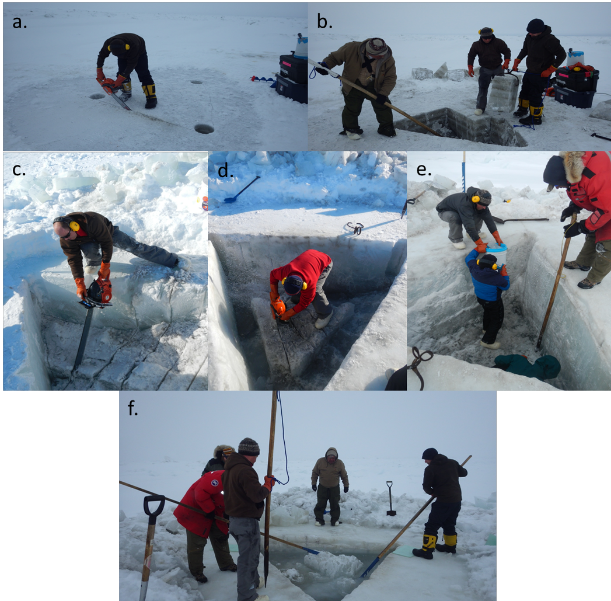
Figure 10.2. Photographic summary of ice removal procedure to create holes for dive access. A triangular shape is outlined on the ice and then blocks cut with chain saws are removed layer by layer (a–e). Once the hole fills with water and the bottom later is cut free with hand saws, the floating block is cut apart and removed (f).
