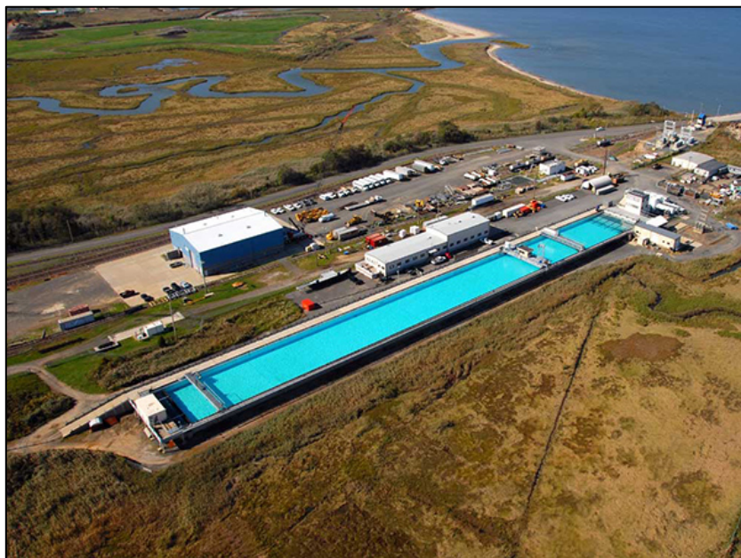
Figure 6. Oil and Hazardous Materials Simulated Environmental Test Tank, Leonardo, NJ
