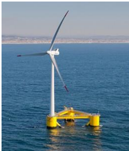
Full-scale prototype of WindFloat device.
