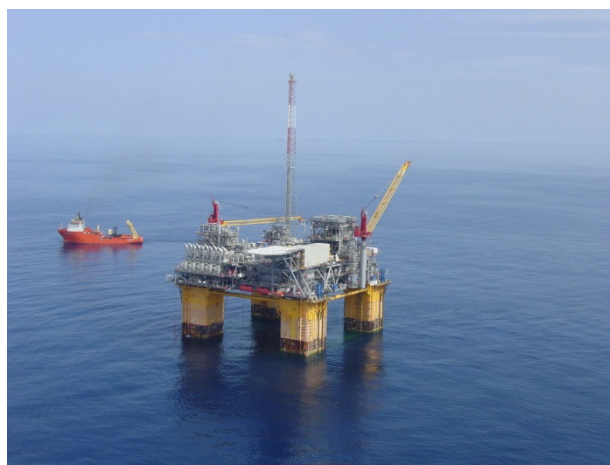
The Na Kika platform in deepwater Gulf of Mexico
