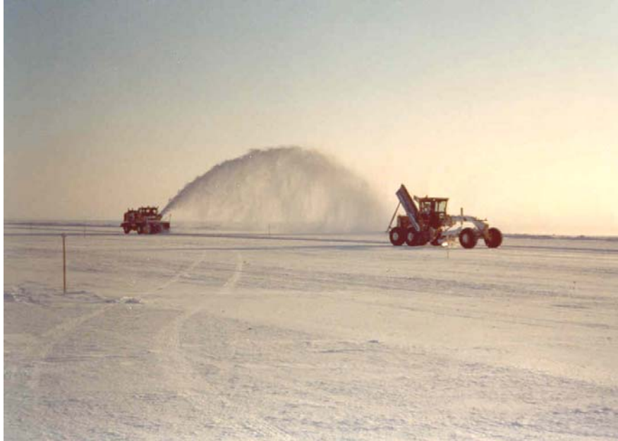
Road Maintenance (grader followed by a snow blower)
