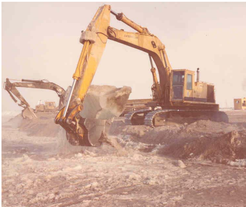
Backhoes catch cut ice blocks out of the water
