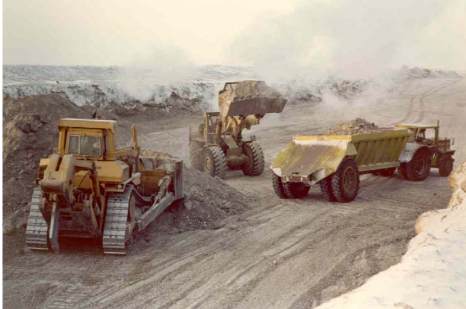
Loading Gravel Trucks at Pit Site
