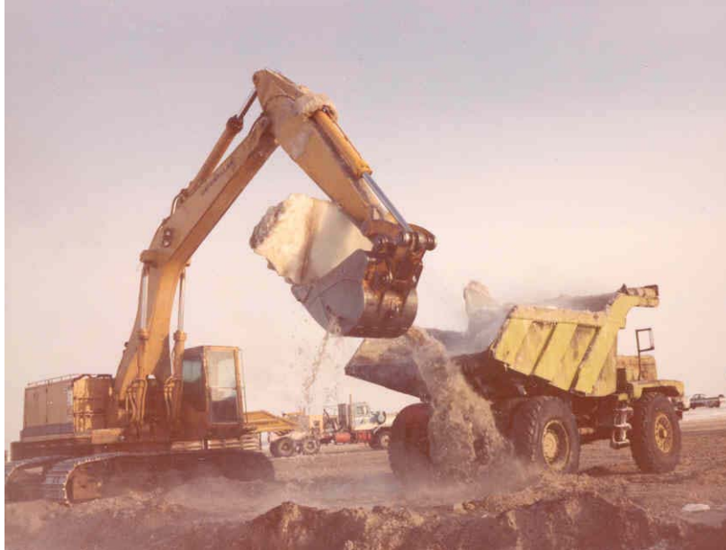
Ice blocks loaded on end dump trucks
