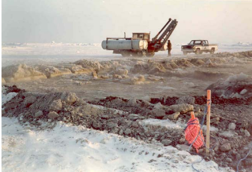
Gravel is pushed into ice hole using dozers
