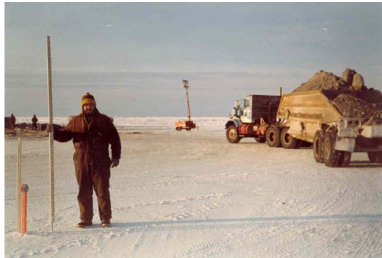
Deflection measurements with level and rod
