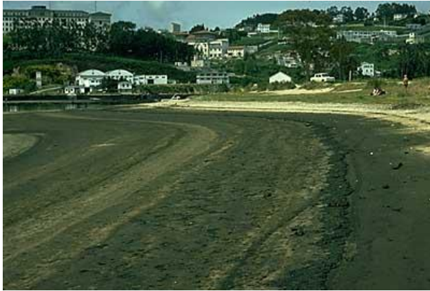
Figure A2: Broken Shoreline Cover
