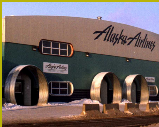
Barrow air passenger terminal
