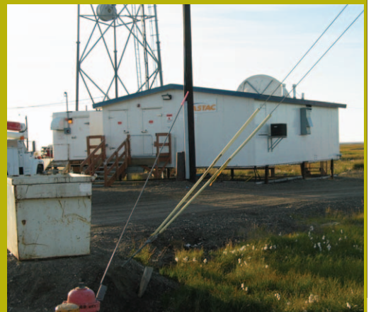
Arctic Slope Telephone Association Cooperative
