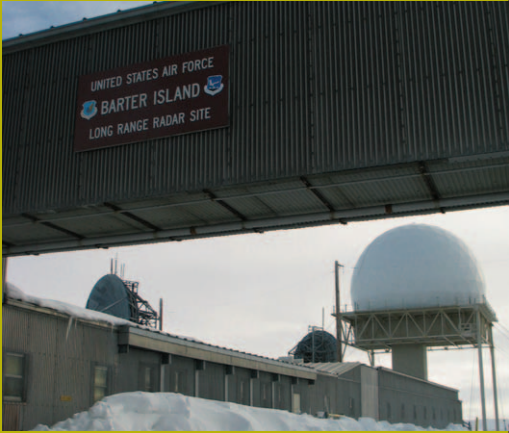
Local DEW Line site
