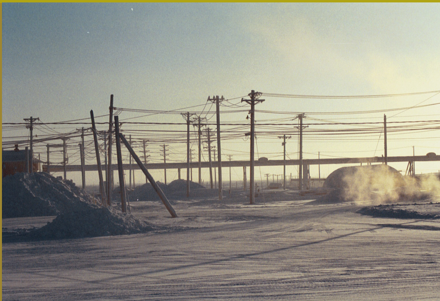
Power lines built by the U.S. Navy are used by Barrow Utilities and Electric Cooperative
