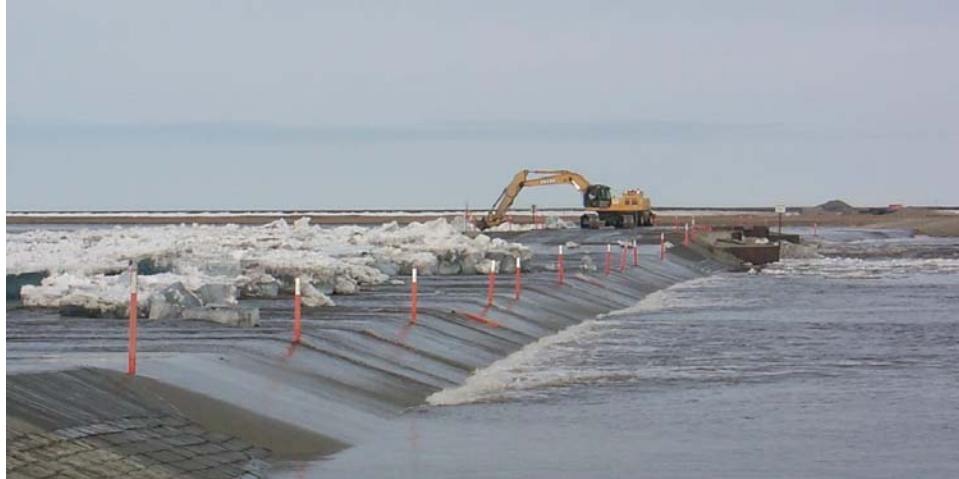
Figure 3-3. Peak flow in the east channel of the Kuparuk River in 2006 creates an overflow of ice and water on the causeway and bridge.
