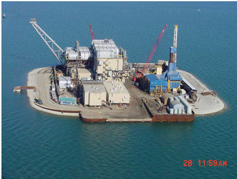
Figure 1-2. The Northstar Development on an artificial island in Alaska State waters.
