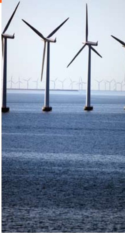
Wind turbines near Copenhagen, Denmark. Stock photo courtesy of Schatz Publishing.
