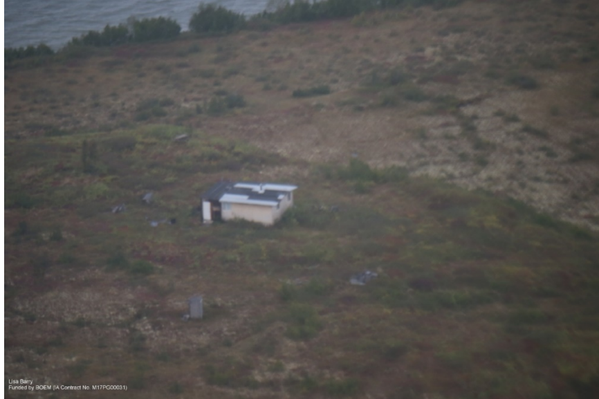
Figure G-1. Aerial view of the cabin located approximately 60 km north of Inuvik, Northwest Territories, Canada, used for the ASAMM Twin Otter FOV target in August 2019.
