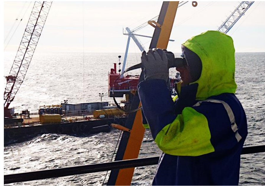
Protected Species Observer (PSO) Block Island Wind Farm Foundation Installation
