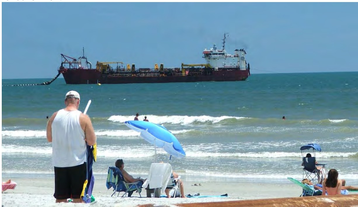
Figure 2. Hopper Dredge with Shore-connected Pipeline During the 2011 Renourishment.
