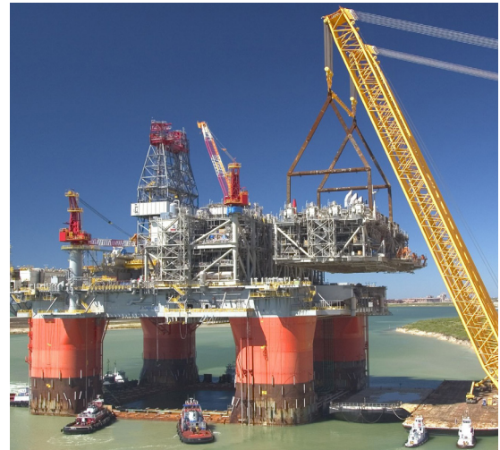
Construction of an oil platform in the Gulf of Mexico
