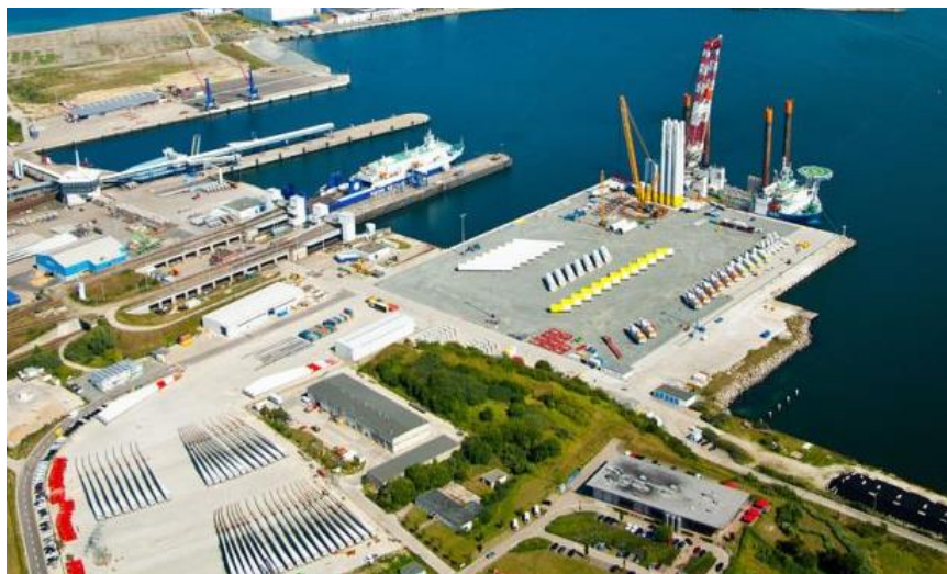
Figure 7: WTG Pre-assembly Harbour Baltic 2 4
