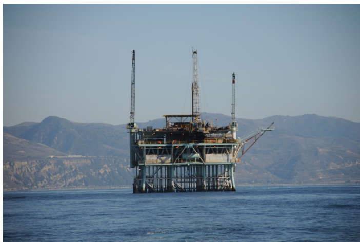
Carpinteria platform offshore California
