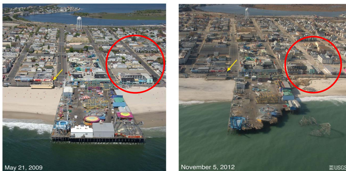
Figure 6.3. Before and After Hurricane Sandy Storm Damages (Seaside Heights, NJ).
