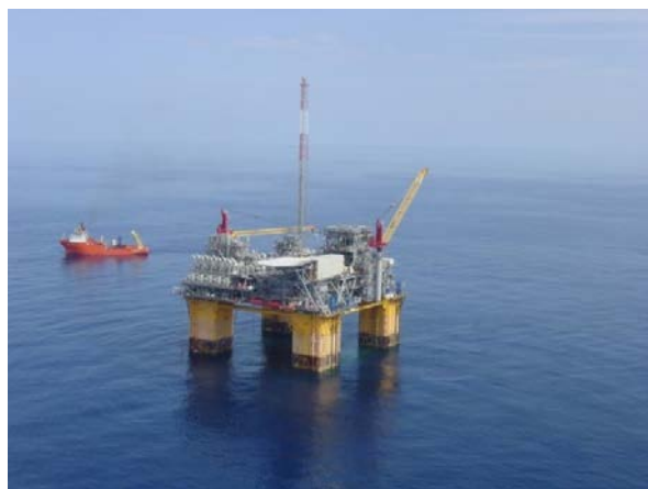
The Na Kika platform in deepwater Gulf of Mexico
