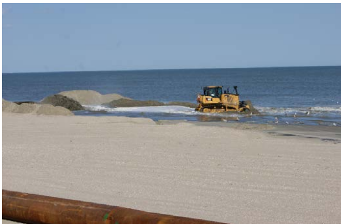
Sand placement work NASA Wallops Island Flight Facility, Virginia
