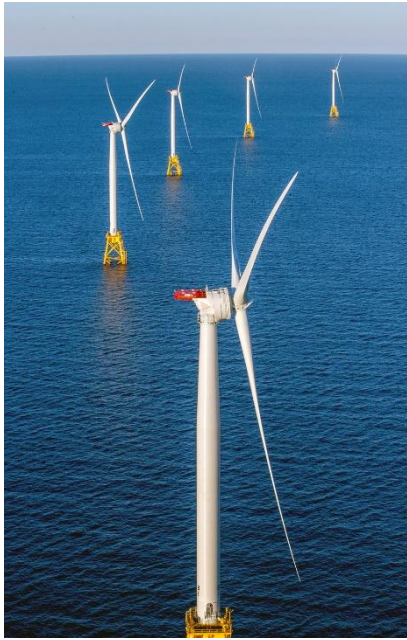
Block Island Wind Farm ( Deepwater Wind )
