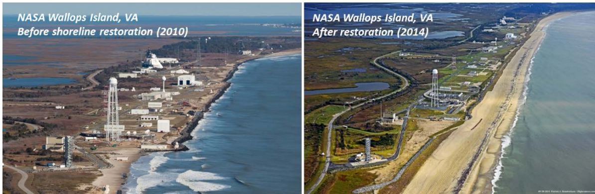
Figure 11. NASA's Wallops Island Flight Facility before and after restoration
