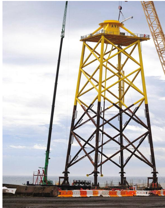
Figure 4.1: Jacket Foundation. Source: Alpha Ventas
