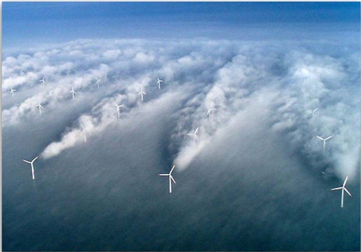
Figure 3-1. Condensation in the Turbulence Field of Wind Energy Turbines
