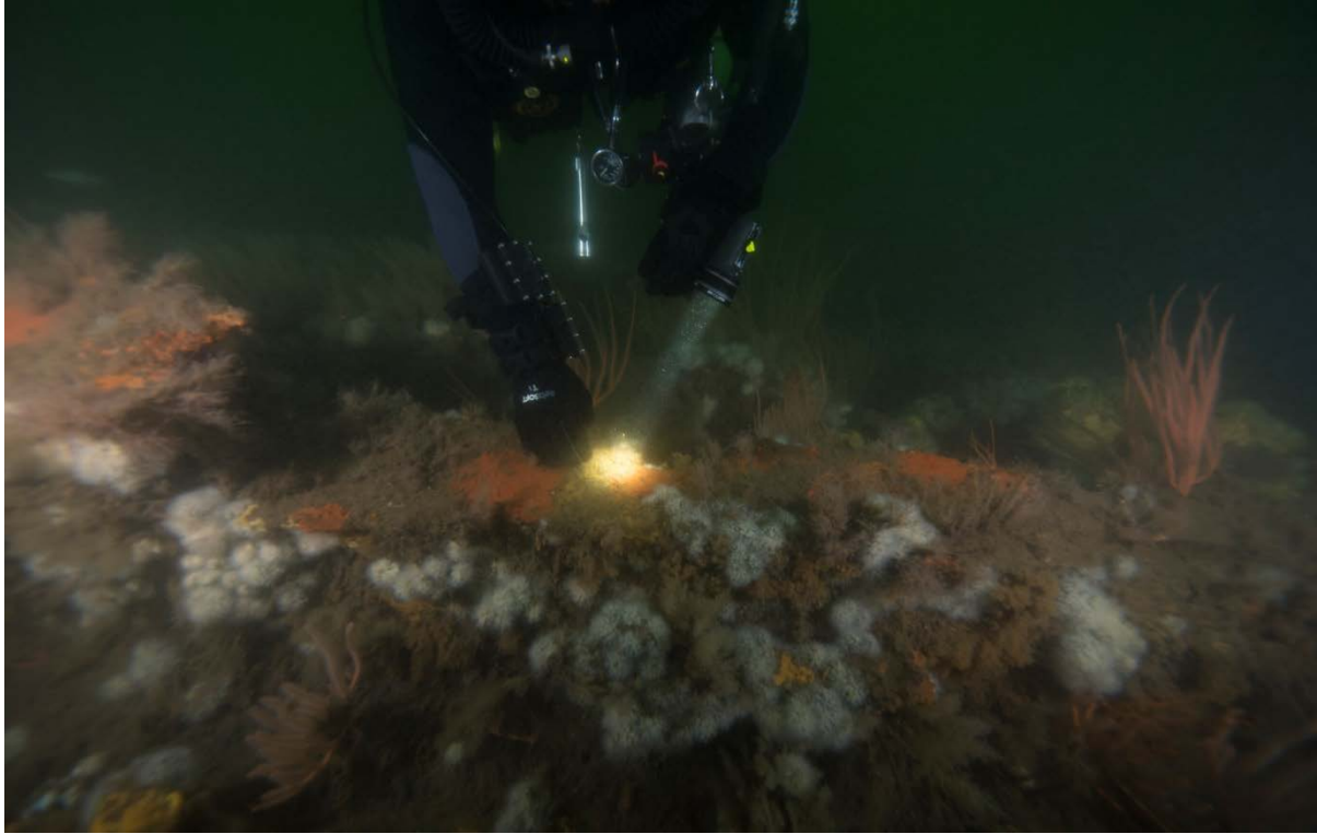
Figure 28. Diver inspecting hull structure at Target 071.
