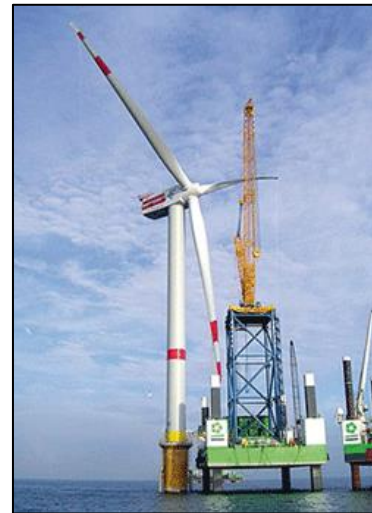
Figure 12. Wind Turbine. Source: BOEM
