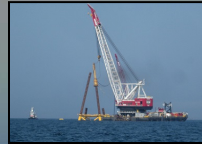
Construction: Drilling and Pile Driving
