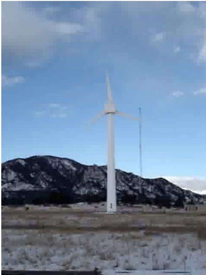
15 Meter Diameter and 100 kW PhotoCredit: Robert Thresher, NREL
