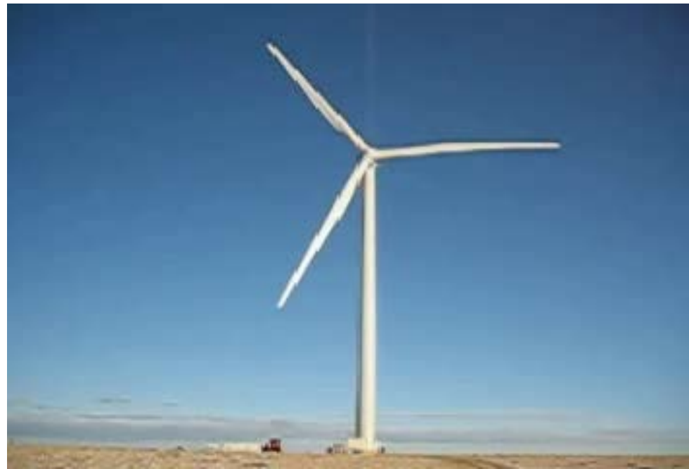
Clipper 2.5MW wind turbine. 93 Meter Diameter Photo Credit: Alan Laxson, NREL
