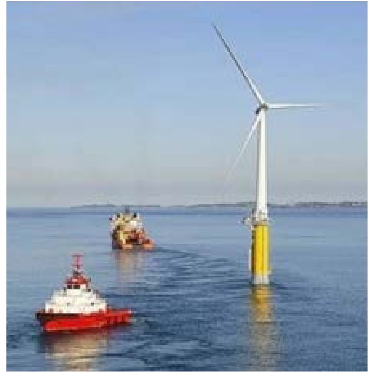
2.3 MW Statoil Floating Turbine in 2009
