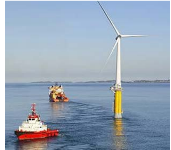
2009 Statoil HyWind Turbine Load-out
