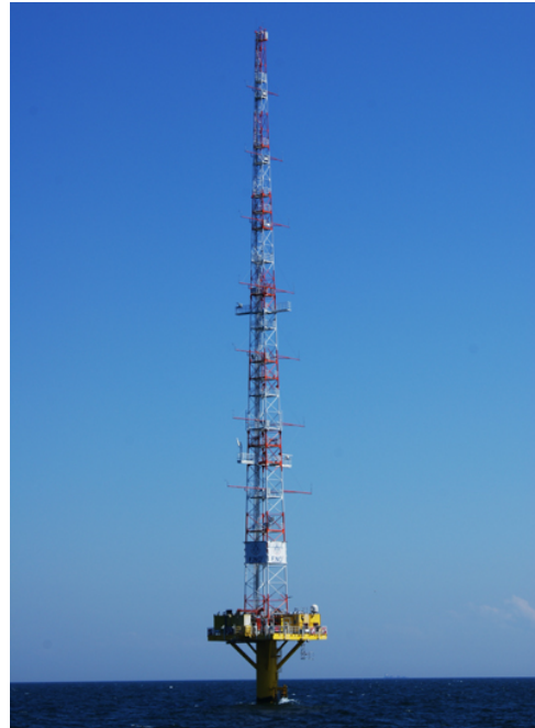
Figure 3-2 Example of a Lattice Mast Meteorological Tower with a Monopile Foundation
