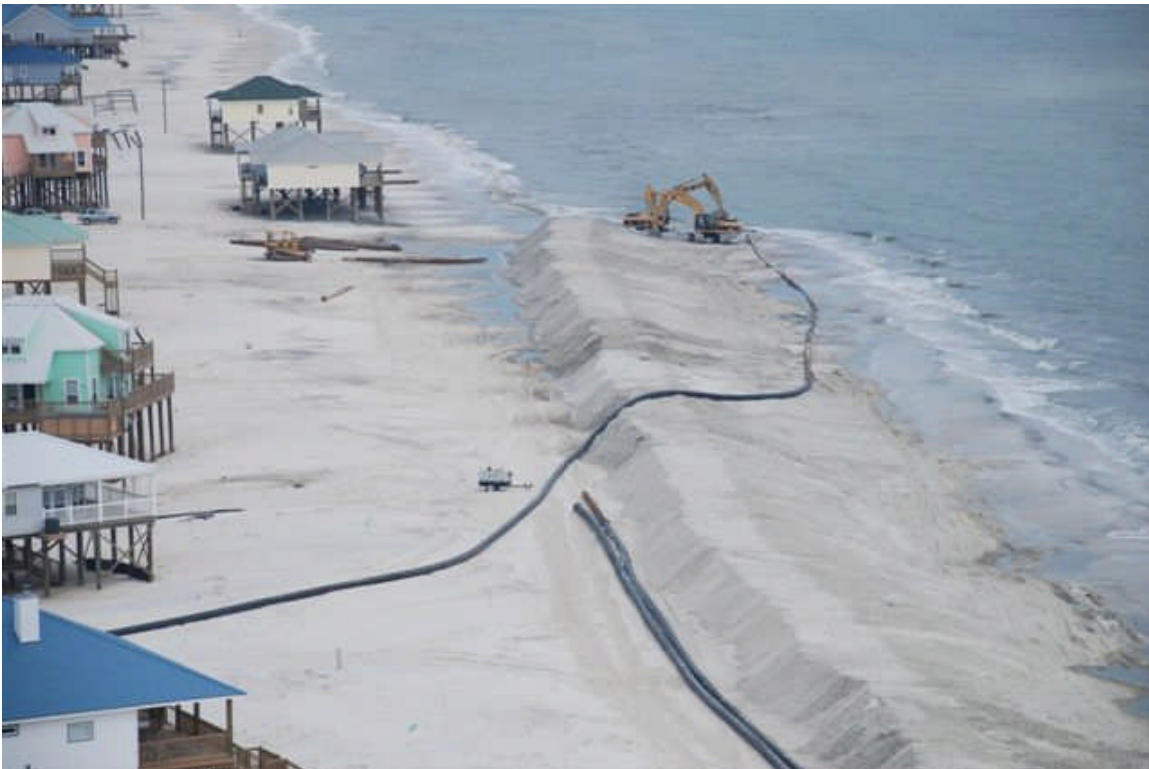
Figure 6.--Dauphin Island Emergency Berm construction.
