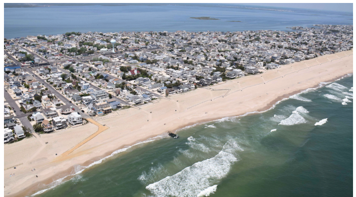
The Long Beach Island project completed in November 2016. Photo by the U.S. Army Corps of Engineers.
