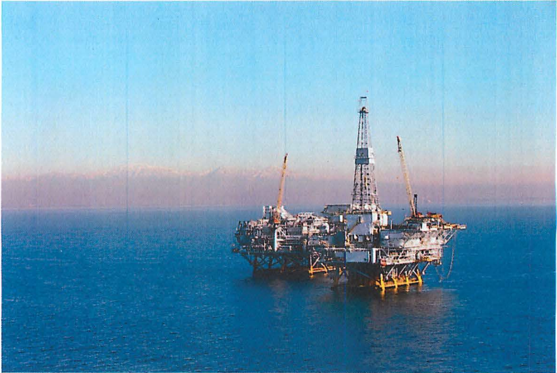
Platforms Ellen (foreground) and Elly
