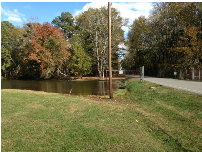
Same view as in previous picture moving eastward toward Lake Christine. Note small wetland fringe at edge of lake. Upland road shoulder to wet fringe.
