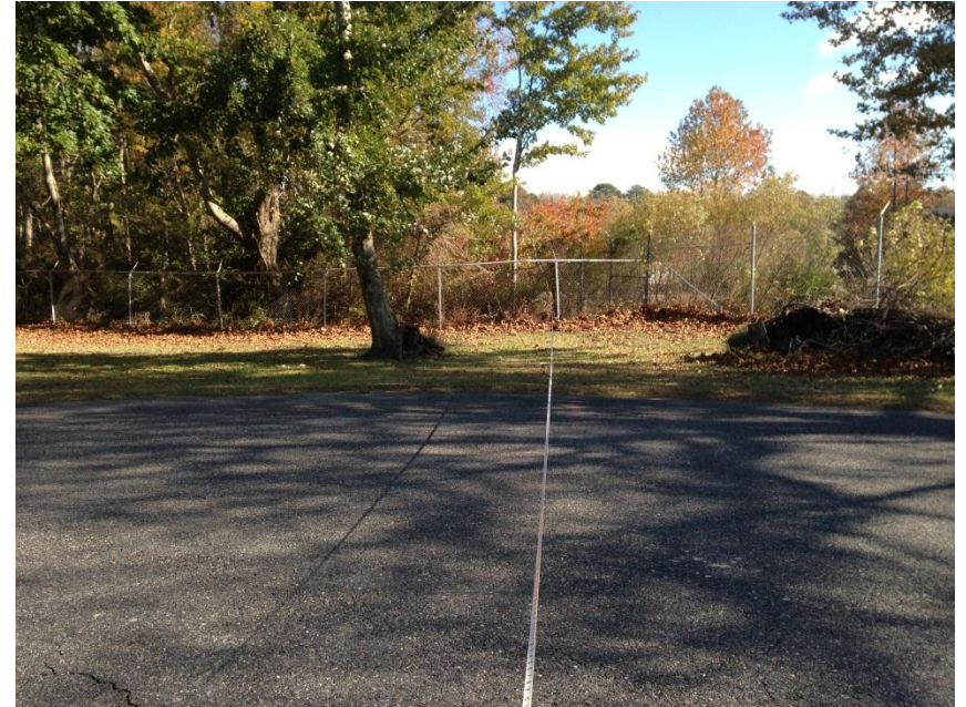
View east from near the south end of the proposed interconnect station area at intersection of unnamed road and S. Birdneck Rd. Tape measures 70 feet from edge of unnamed road pavement across the paved arc toward the fenceline.
