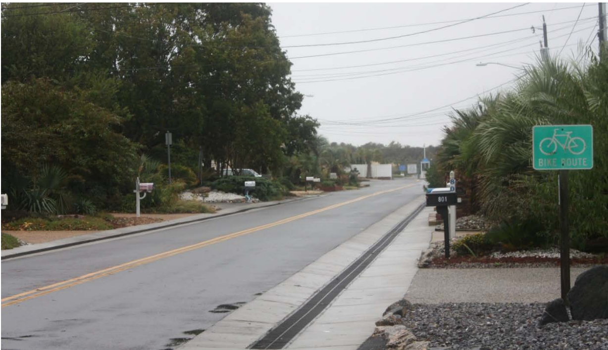
Photo 7. Looking southeast along Vanderbilt Avenue toward the Alternative 2 Switch Cabinet location. The cabinet was planned for the area behind the fence and foliage at the center of the photograph. (James Sexton, Tetra Tech, October 11, 2013)
