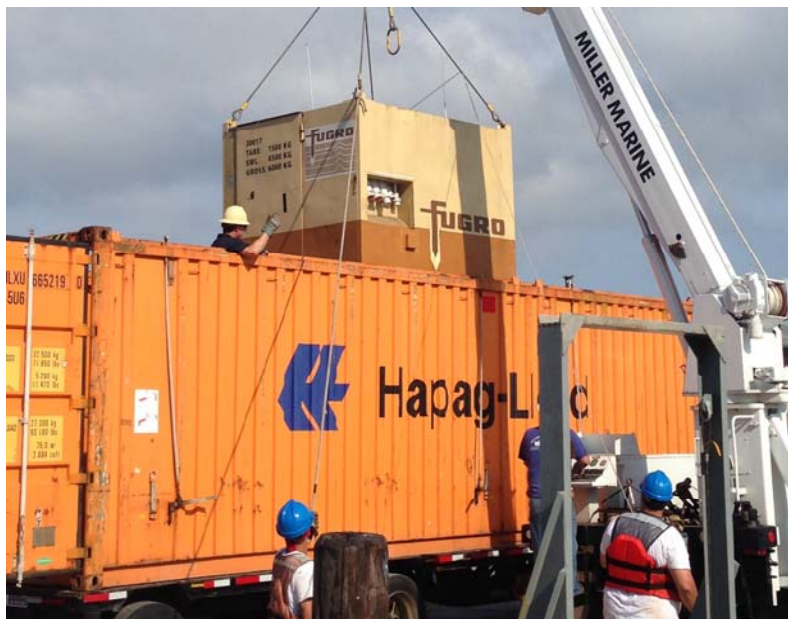
Mobilization of PCPT Data Acquisition System
