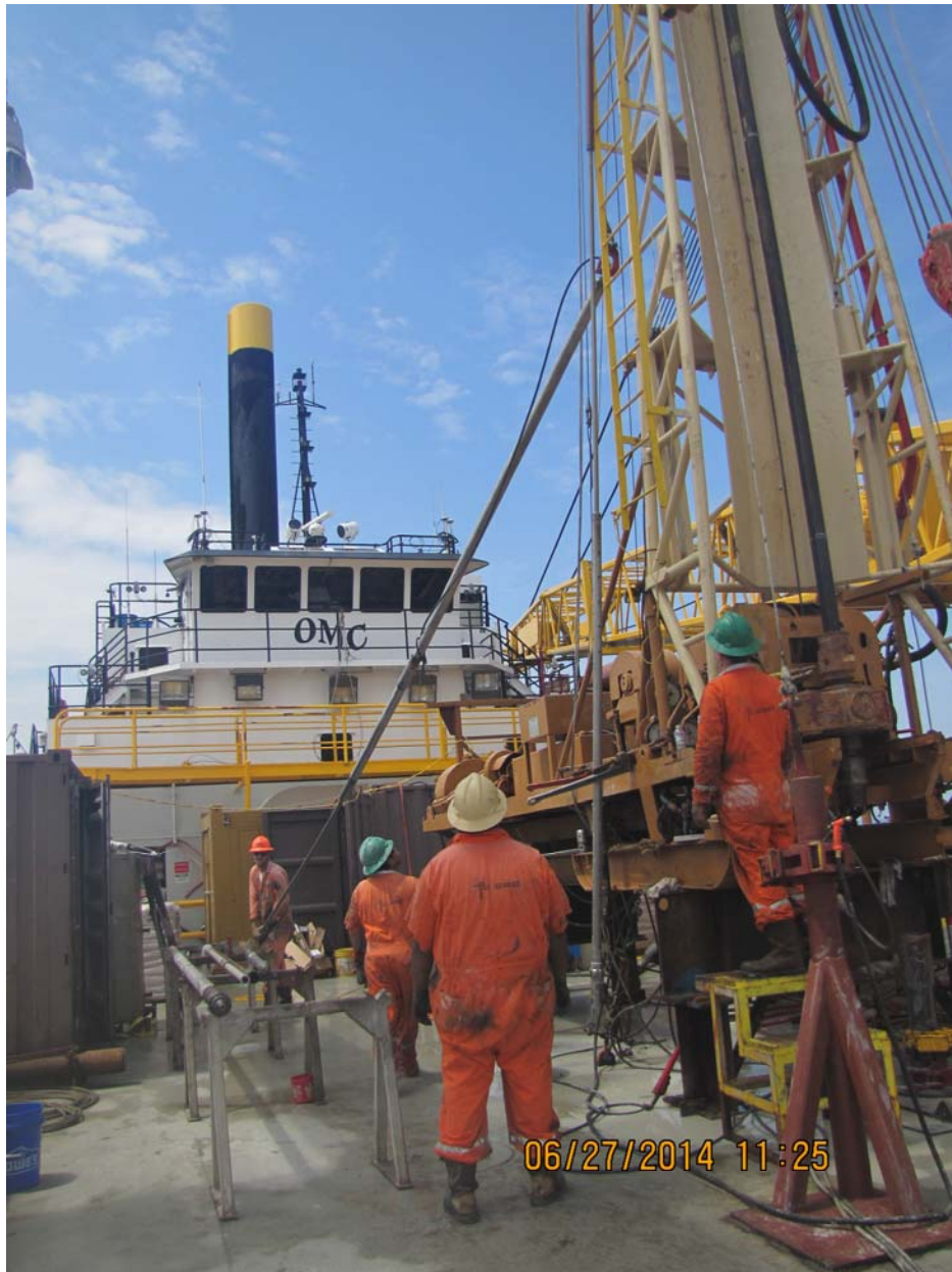
Disassembling Rods during Drilling Operations
