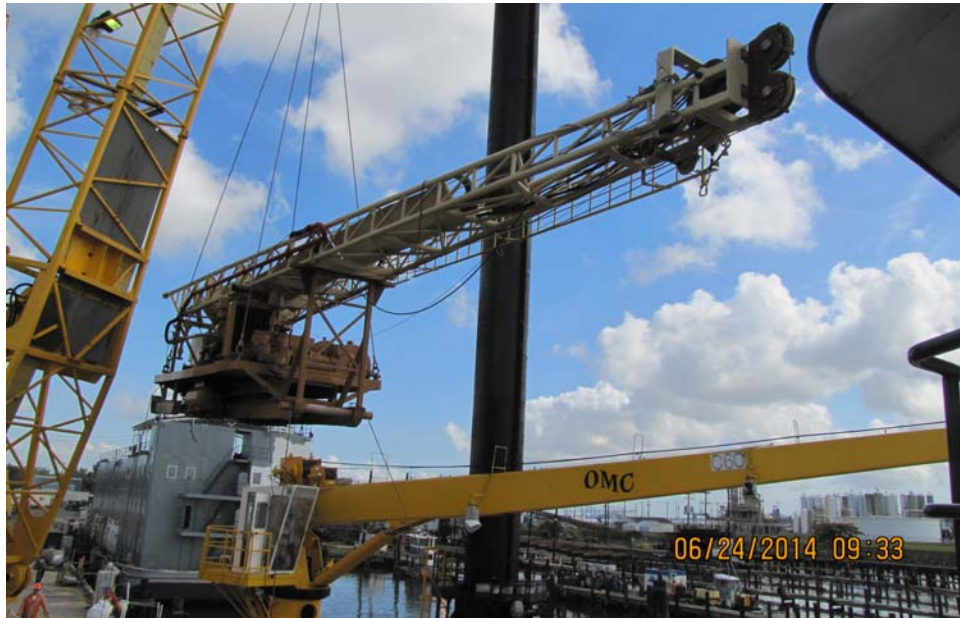
Mobilization of Failing DMX 1500 Drill Rig
