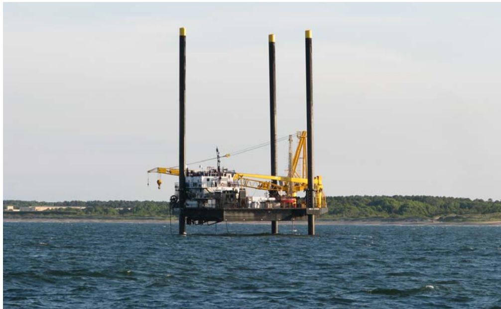
The Inez H. Eymard Jacked Up and Drilling at NB-11
