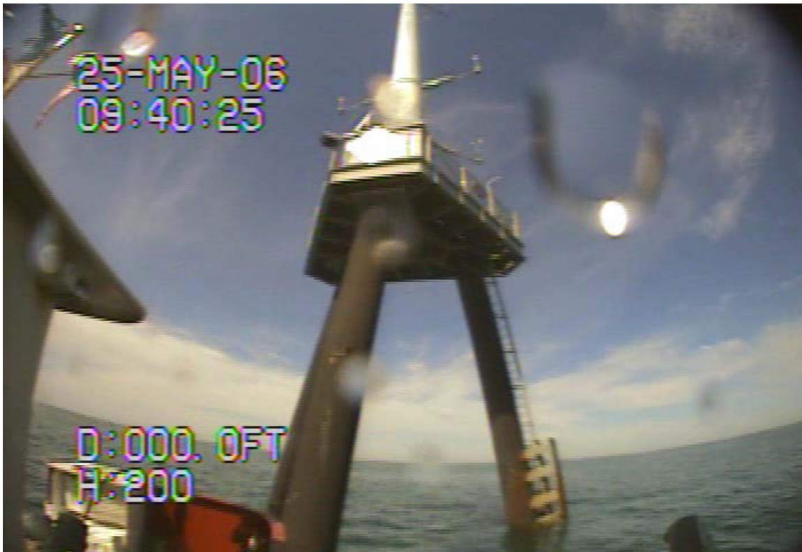
1. View of the MT from the deck of Patriot Too
