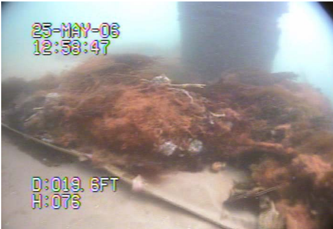
9. Existing mats at base of Southwest pile, Southwest pile in background
