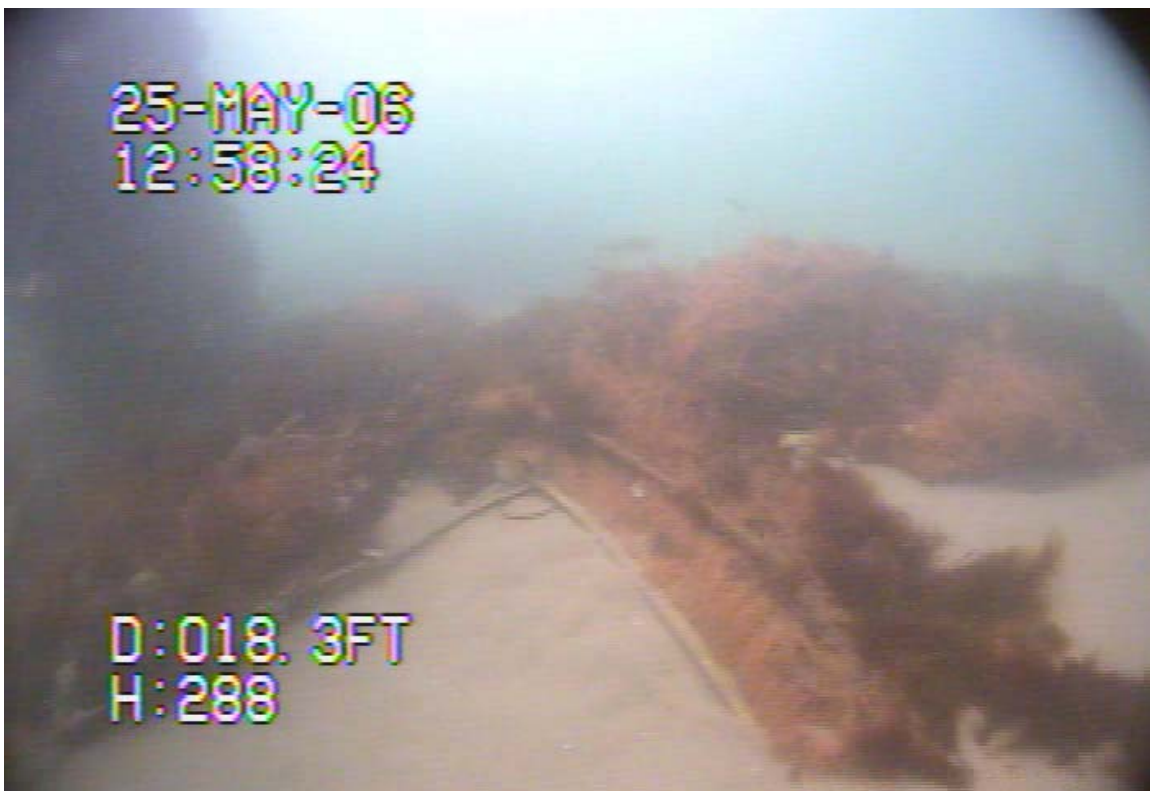
8. Existing mats at base of Southwest pile
