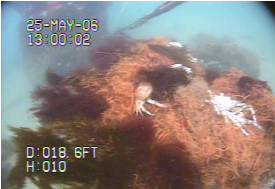
10. Existing mats at base of Southwest pile, Southwest pile in background
