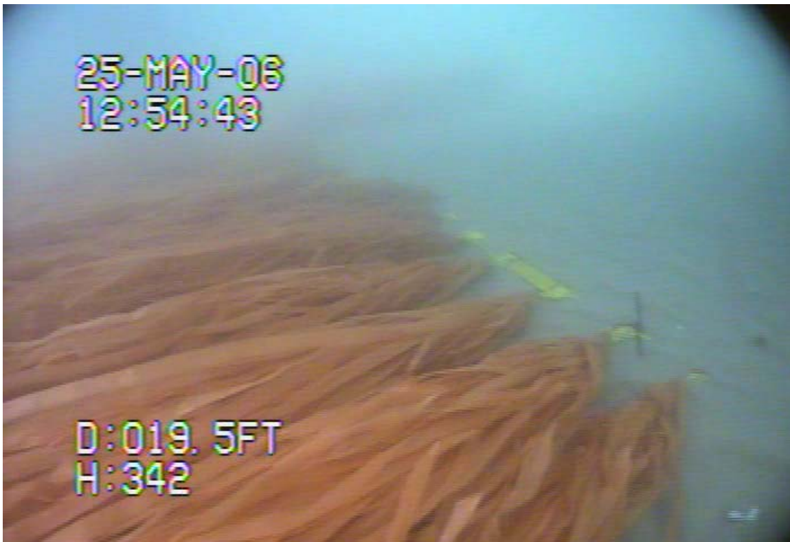
6. Newly installed mats at base of Southeast pile
