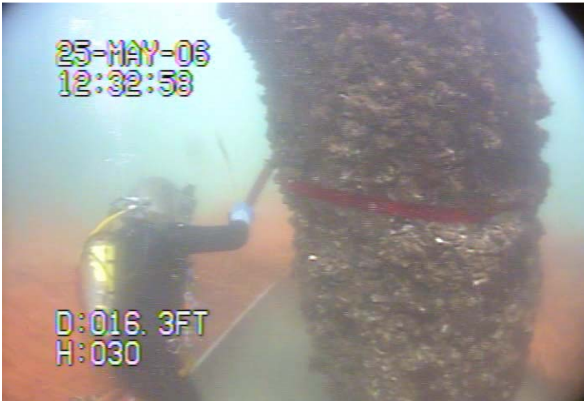
3. Installing ratchet strap on Southeast pile
