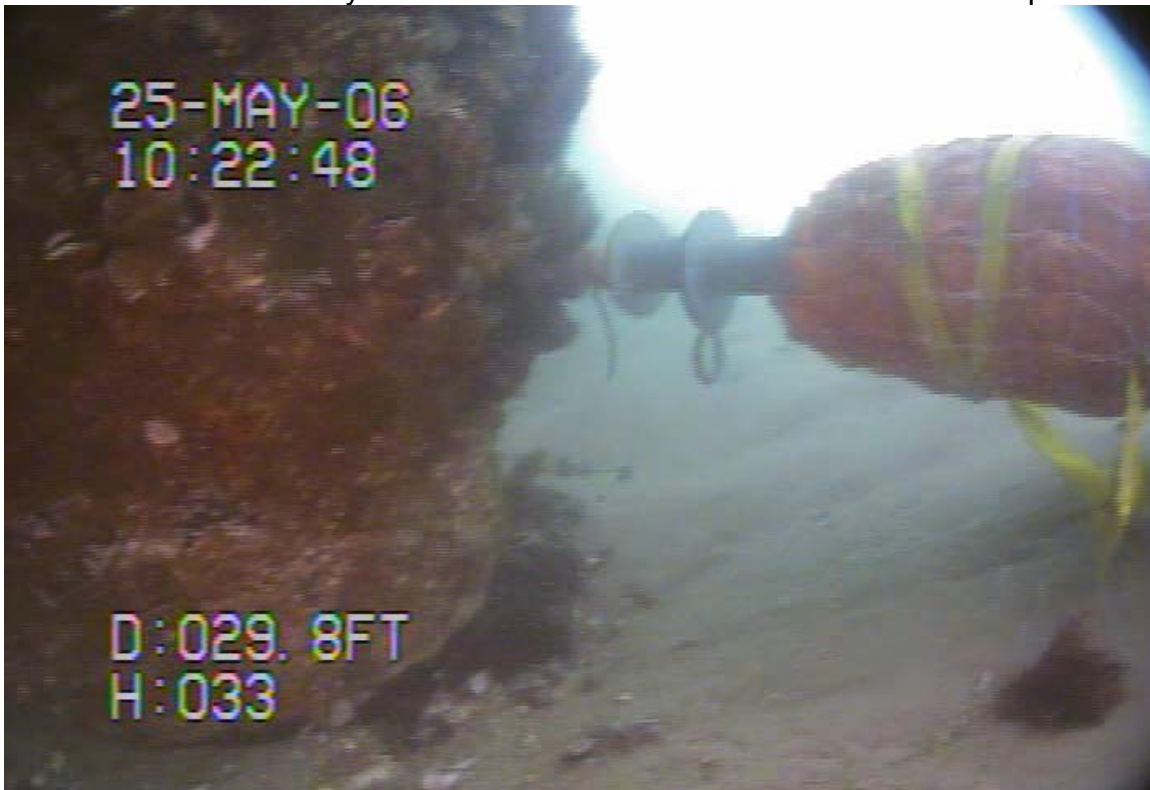
13. Mat on bottom ready for installation and scour at base of Southeast pile
