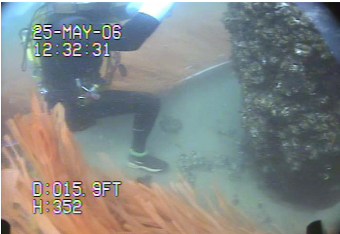
2. Newly installed mats at base of Southeast pile
