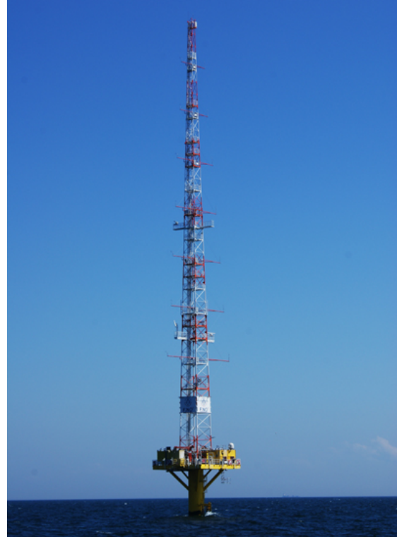
Figure 3-3. Example of a lattice mast meteorological tower with a monopile foundation
