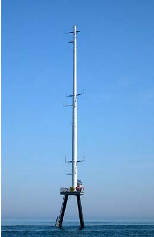
Figure 3-2. Example of monopole mast meteorological tower
