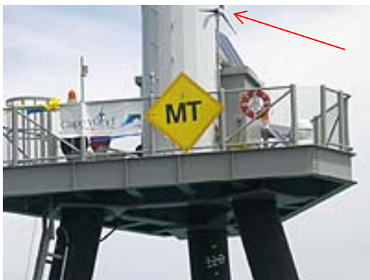
Figure 4.4. Cape Wind meteorological tower platform with a micro wind turbine (see arrow) that has a rotor diameter of approximately four feet.
