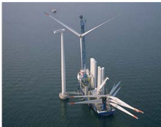
Figure 1. Installation of Shaft, Turbine, and Blades. Source:
