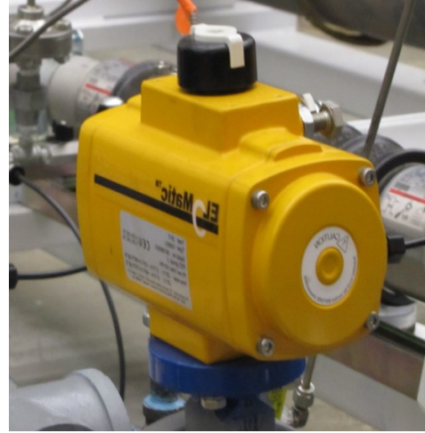
Figure 3.9 Quick closing valve
