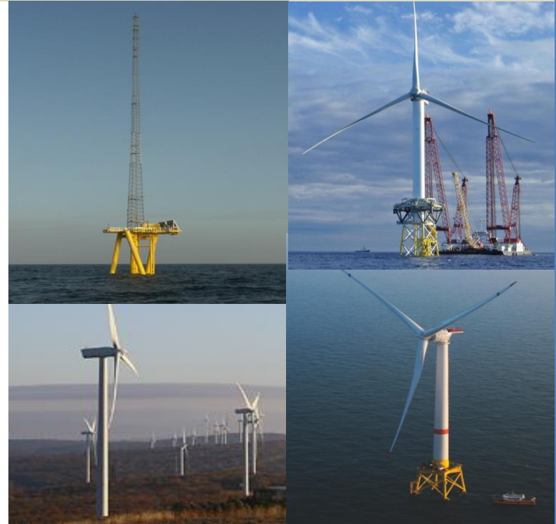
Top left, clockwise: Met tower on Keystone jacket, Beatrice Wind Farm (KBR), Alstom Belwind turbine, Dominion NedPower project
