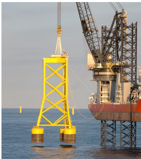
First prototype suction-bucket jacket at Borkum Riffgrund I, pioneered by DONG Energy
